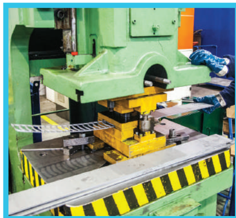
Installation: Mechanical Power Press
